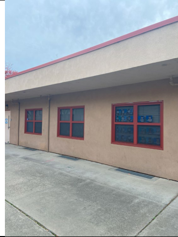
Typical exterior view of the classroom buildings.
