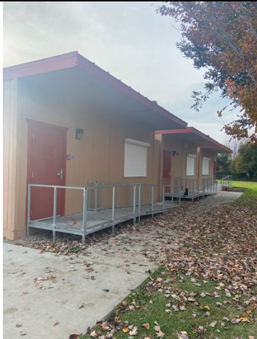
Typical exterior view of the portable classroom buildings.
