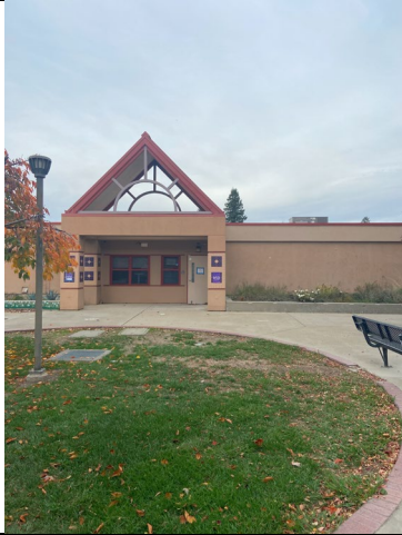
Typical exterior view of the classroom buildings.
