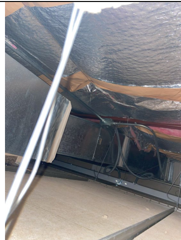
View of the above ceiling spaces within the portable buildings.
