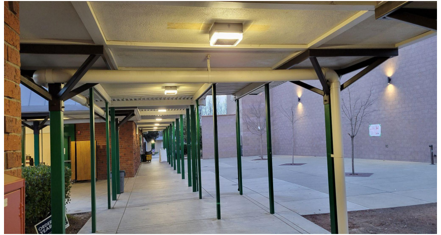
LED Lighting Exterior Retrofit Phase 1 Multi-site
