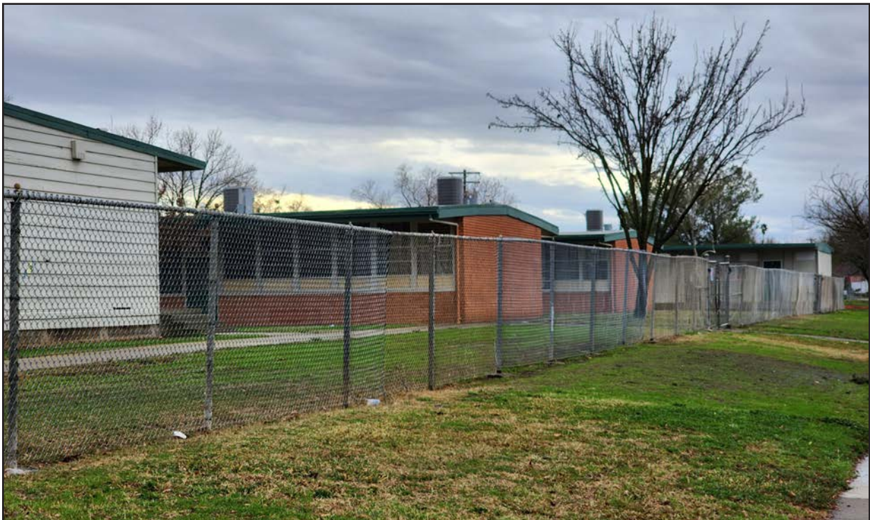
View of Edward Kemble Elementary School.
