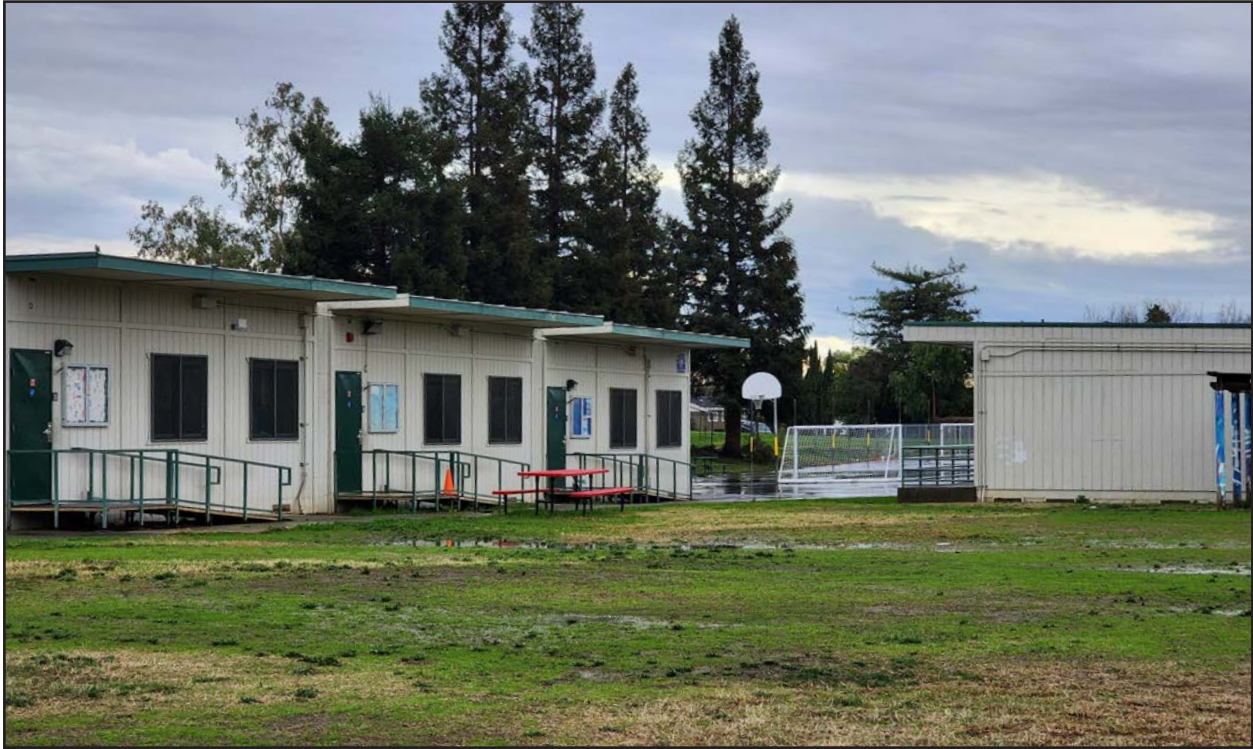
View of Edward Kemble Elementary School.
