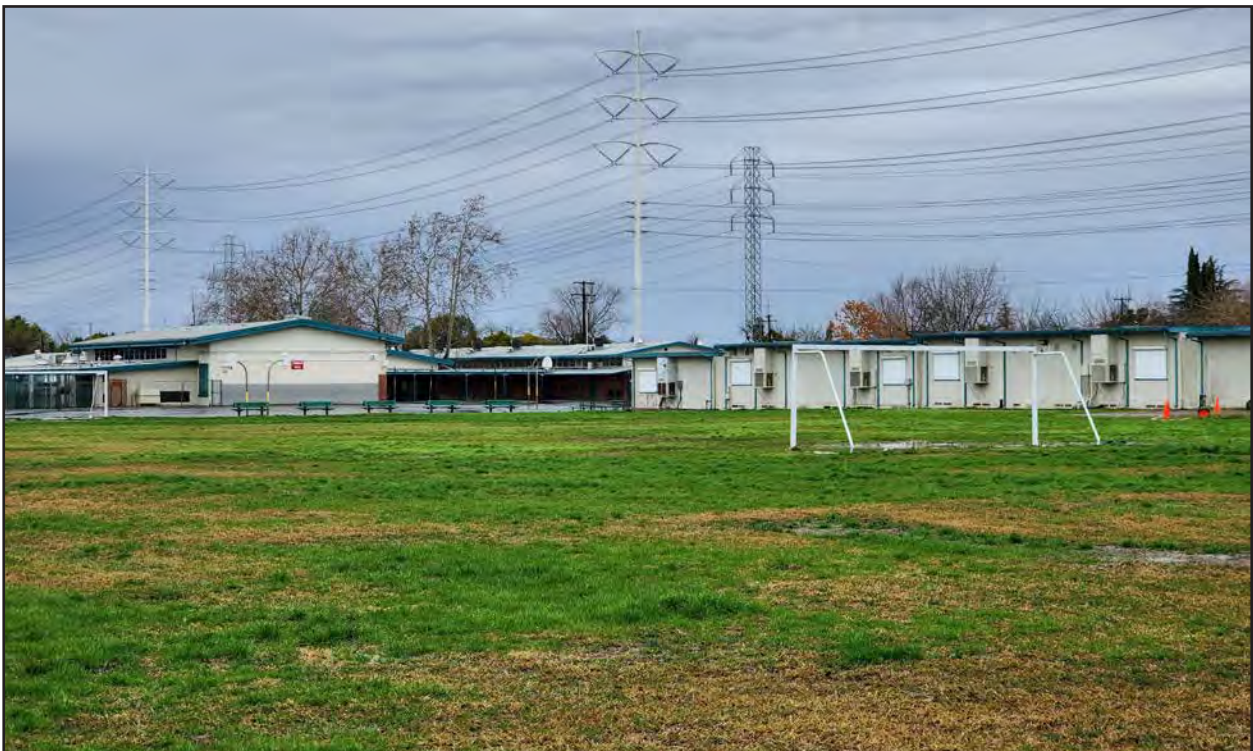
View of Nicholas Elementary School looking southeast.
