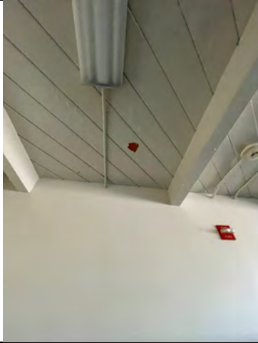
Example of the White paint over Orange paint on the ceilings of Buildings E & F. The paints are lead-based paints.
