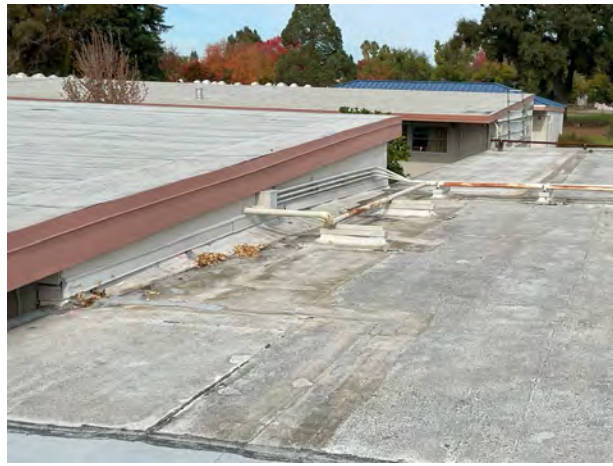
Example of the roofing systems of the school buildings.
