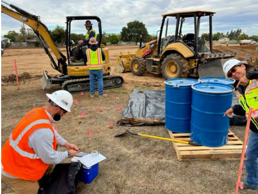
View of excavation location at A-15 with flags marking the previous sample locations – October 25, 2023
