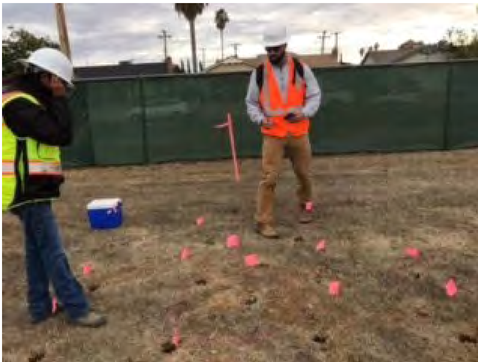
Another view of the excavation location at A-15 – October 25, 2023
