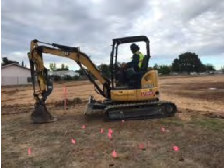
Backhoe ready to start excavation activity on October 25, 2023
